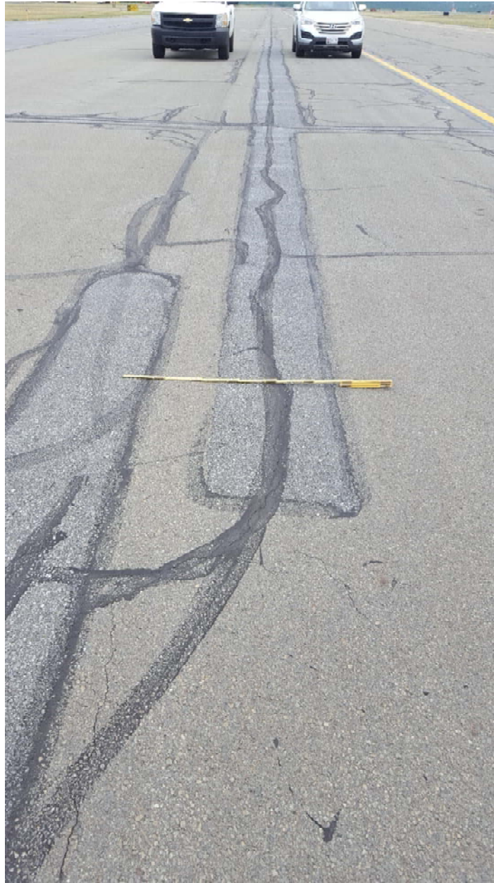
Taxiway B Low Patching
