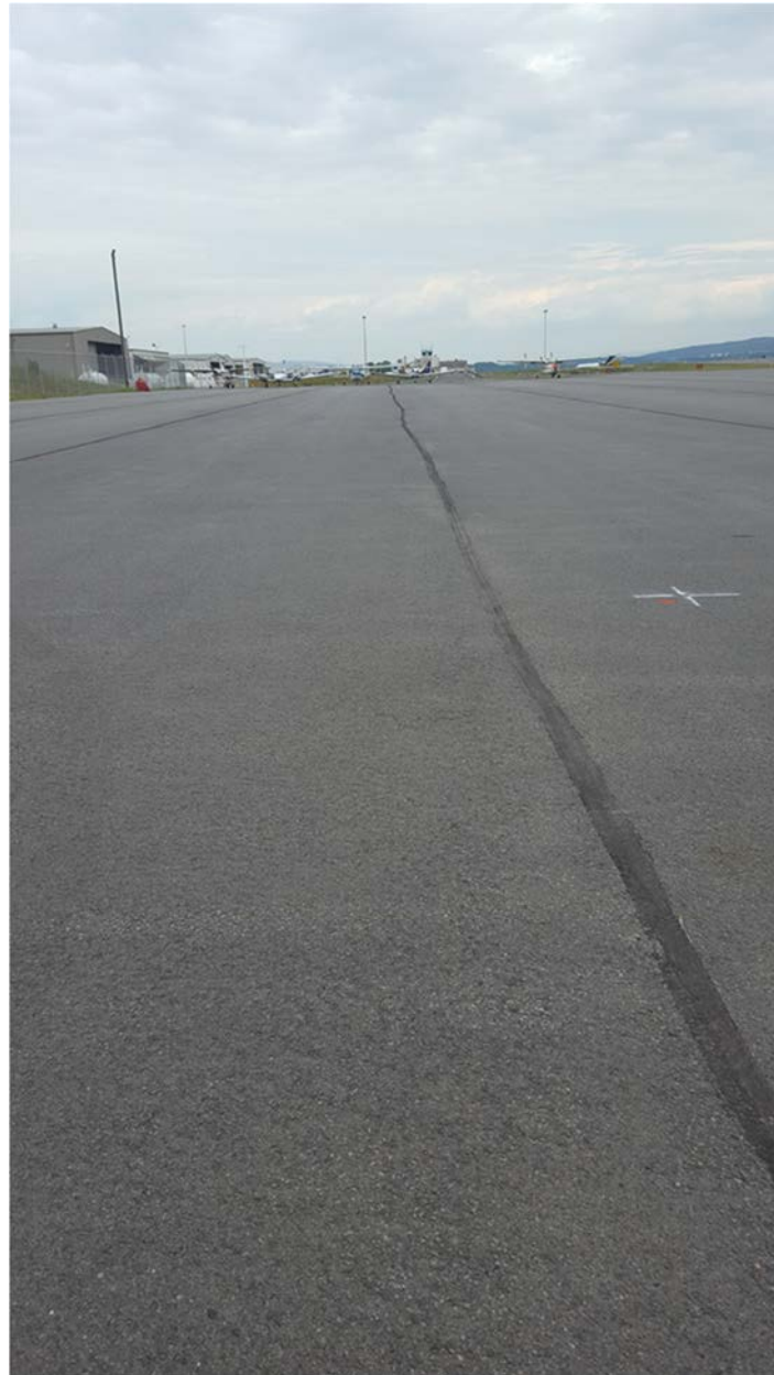
Overall South General Aviation Apron
